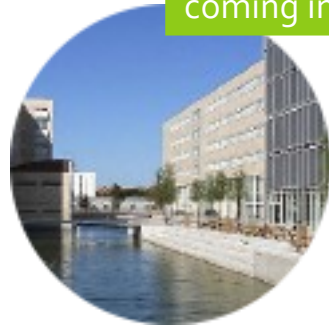
Innovative Rainwater Collection System
